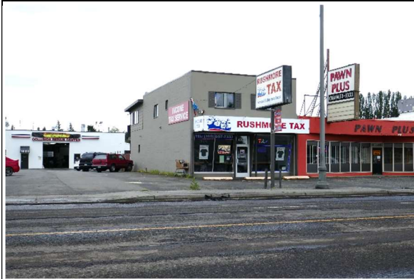
Looking E from State Ave
