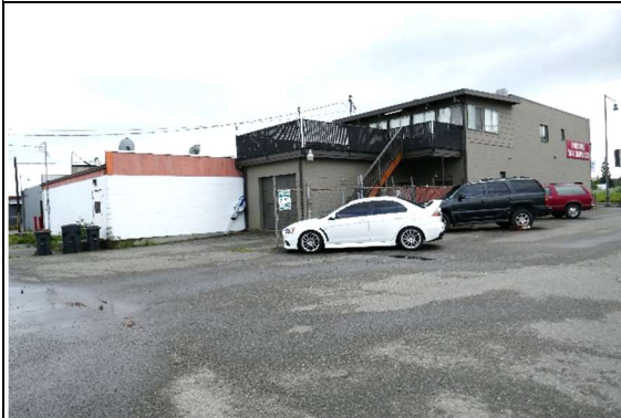
Looking SW at rear of property
