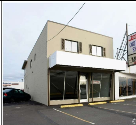
Looking E from State Ave
