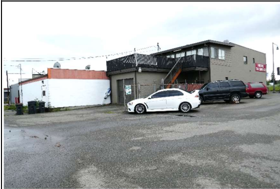
Looking SW at rear of property
