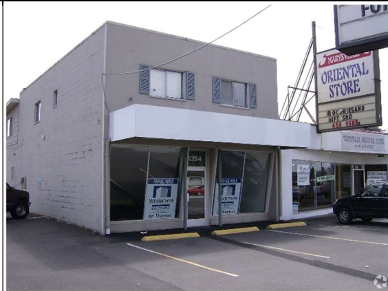
Looking E from State Ave
