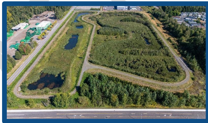
Figure 21. North Marysville Regional Stormwater Ponds
