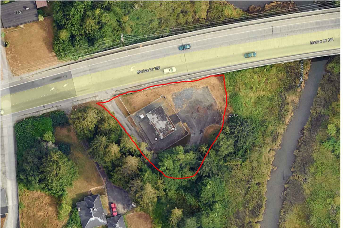
Figure 1 Marysville West Lift Station
