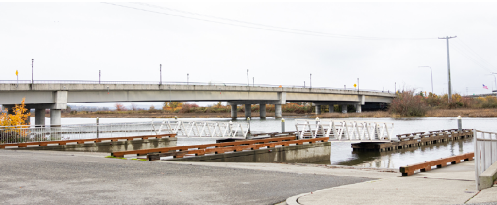
Waterfront access including a boat launch is provided at Ebey Waterfront Park.
