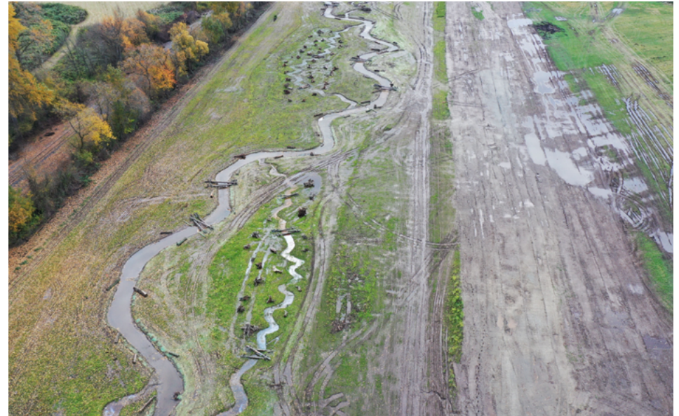
Edgecomb Creek was relocated and reestablished as a meandering stream in 2022. Photo credit: Northpoint Development.
