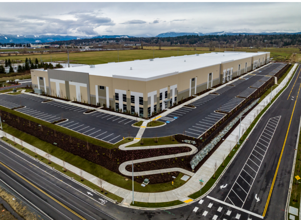
Tesla occupies this new warehouse, the first of nine industrial warehouses planned for the Cascade Business Park. Image Credit: Sierra Construction.
