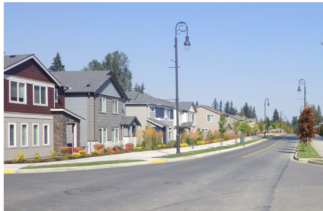
Wide sidewalks, landscaping, and decorative street lighting encourage walking in the East Sunnyside – Whiskey Ridge Neighborhood.
