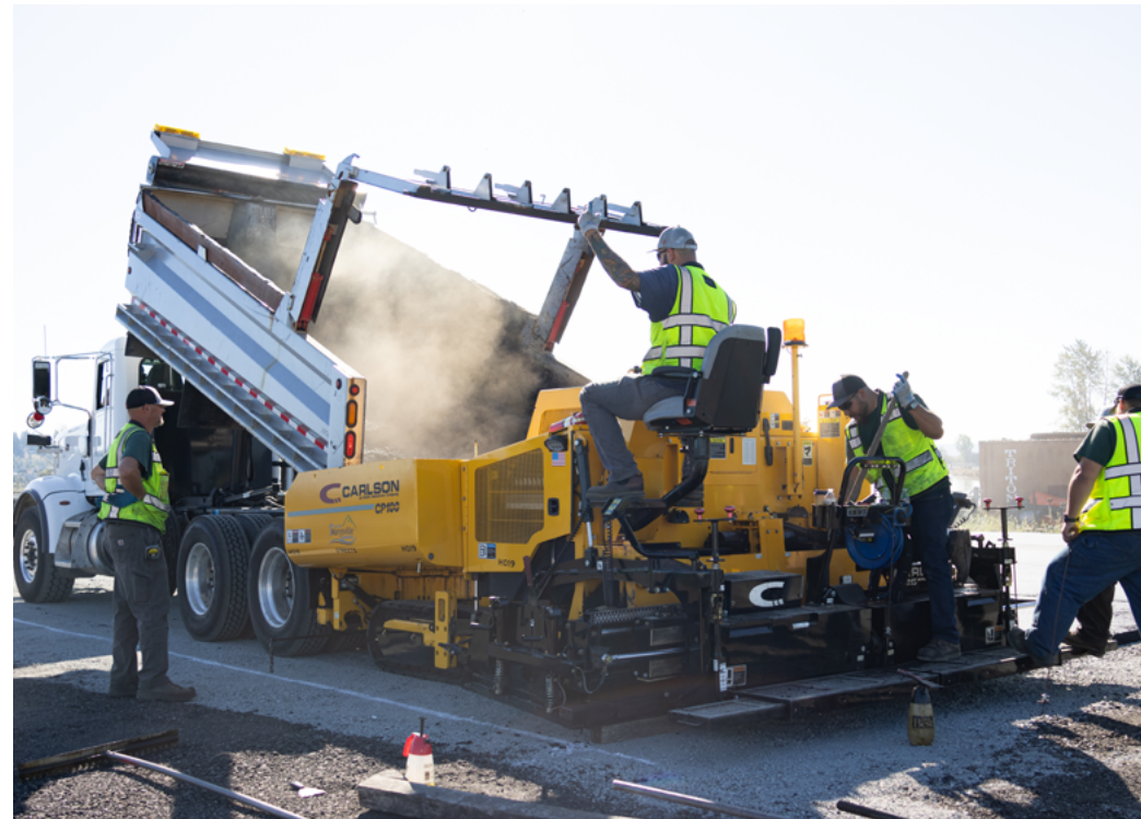
Public Works crews working on a road improvement project.
