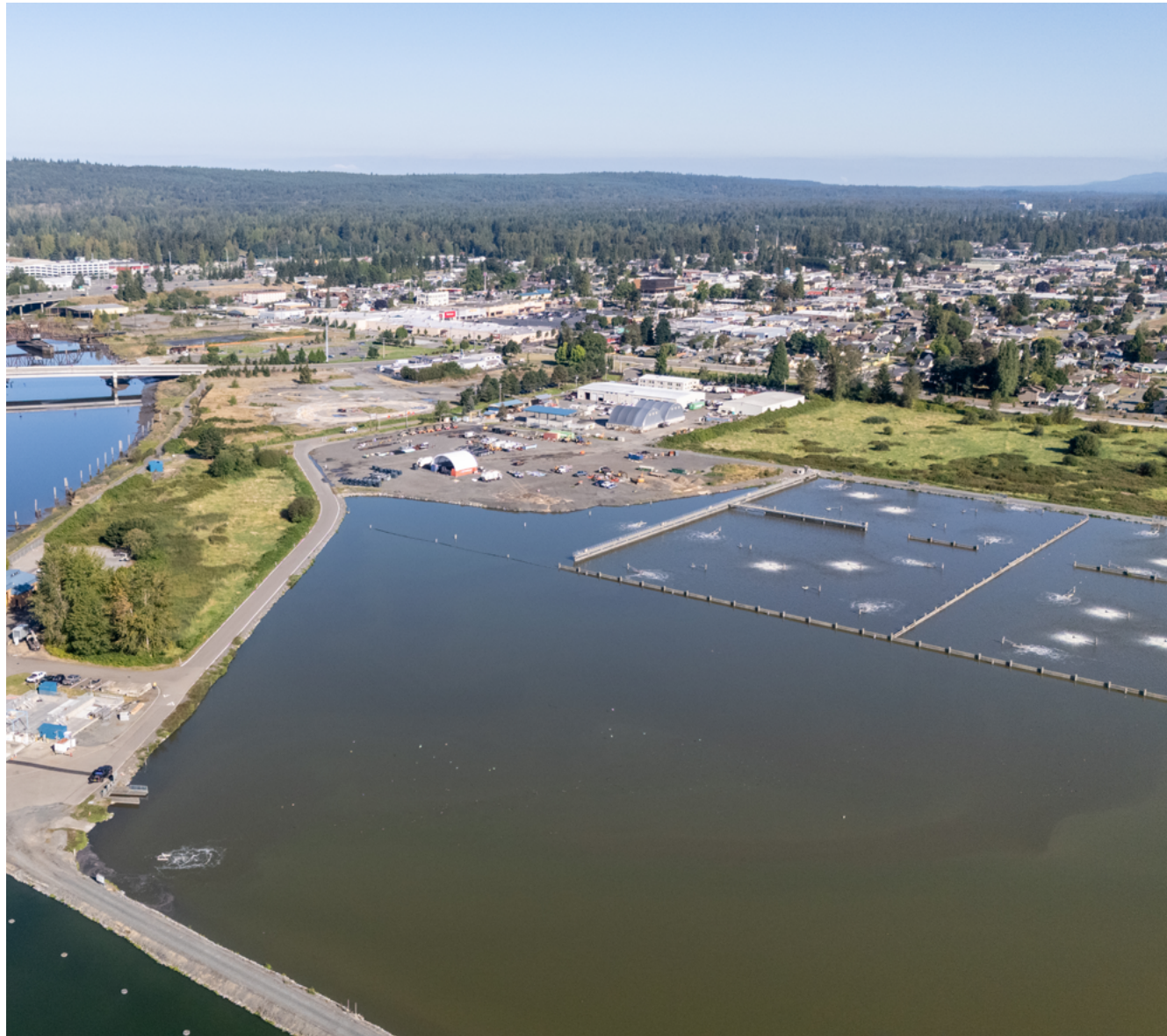
The Marysville Wastewater Treatment Plant is a major capital facility which treats the community's wastewater.
