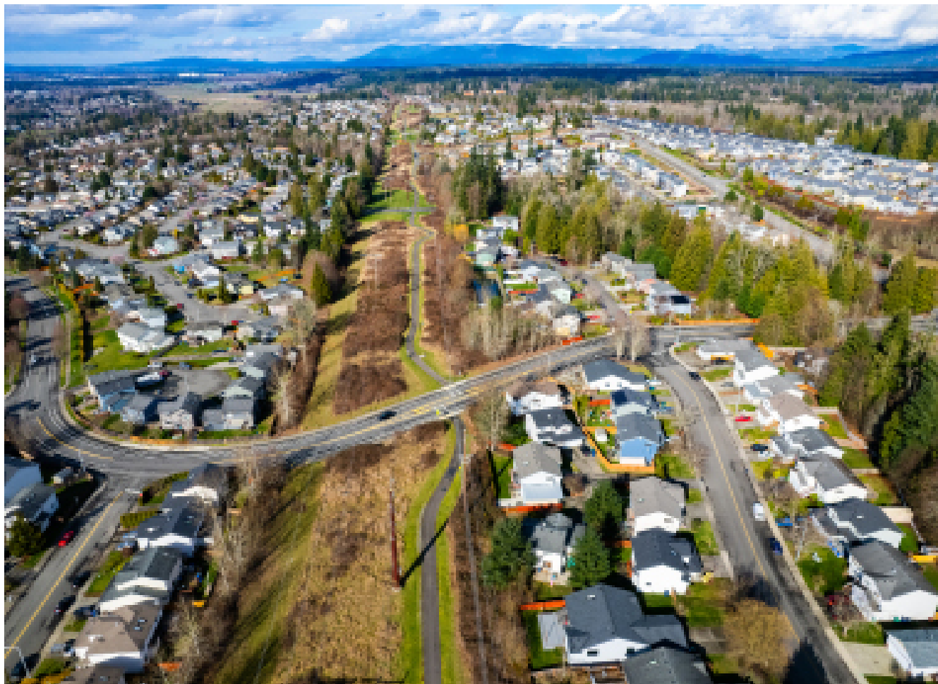
The Olympic Pipeline, Puget Sound Pipeline, and other major regional utilities, are located in the utility corridor shown here.
