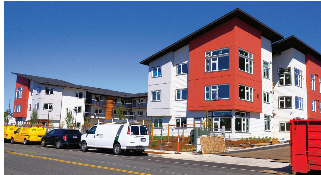
Redevelopment Downtown affords new housing options, but also may result in displacement.
