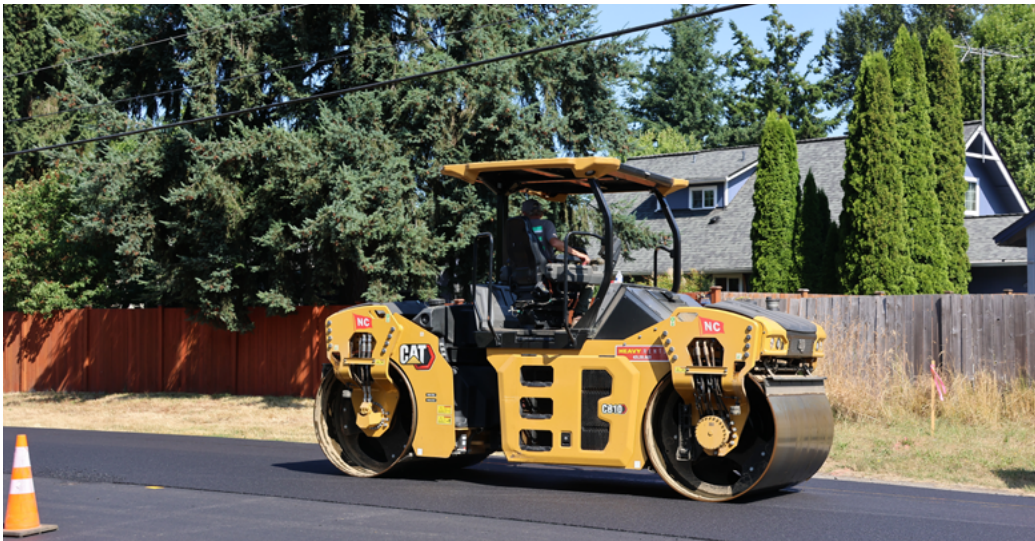
Construction workers repave 132nd Street NE as part of the City's pavement preservation program.
