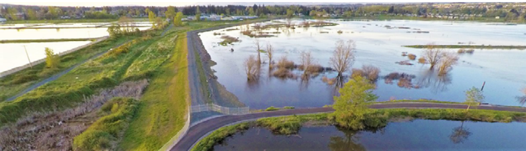
The City received grant funding to increase levee heights to address sea level rise projections, flood mitigation, and estuary restoration.
