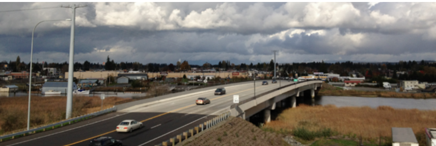
A new I-5 interchange is currently being constructed south of Ebey Slough, which will tie into the SR529 bridge shown here.
