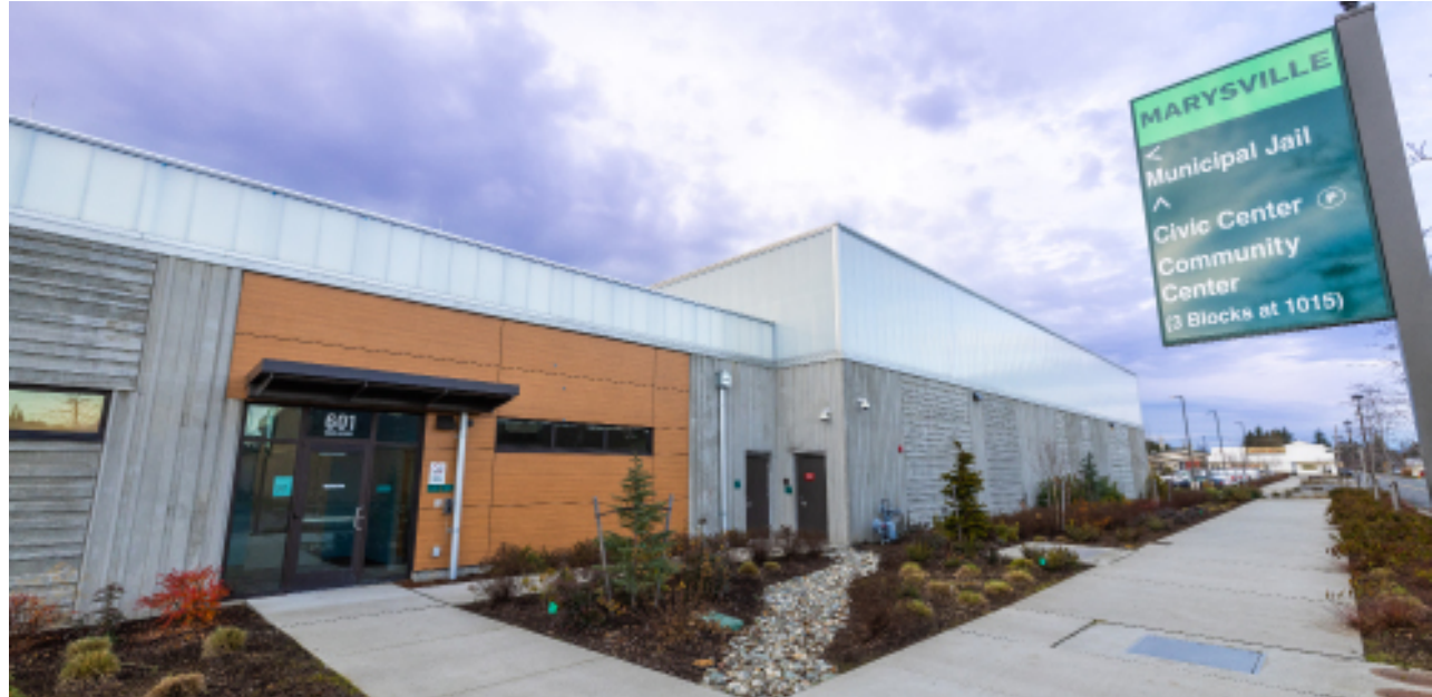
The new Marysville Municipal Jail is an Essential Public Facility that benefits Marysville and surrounding communities.
