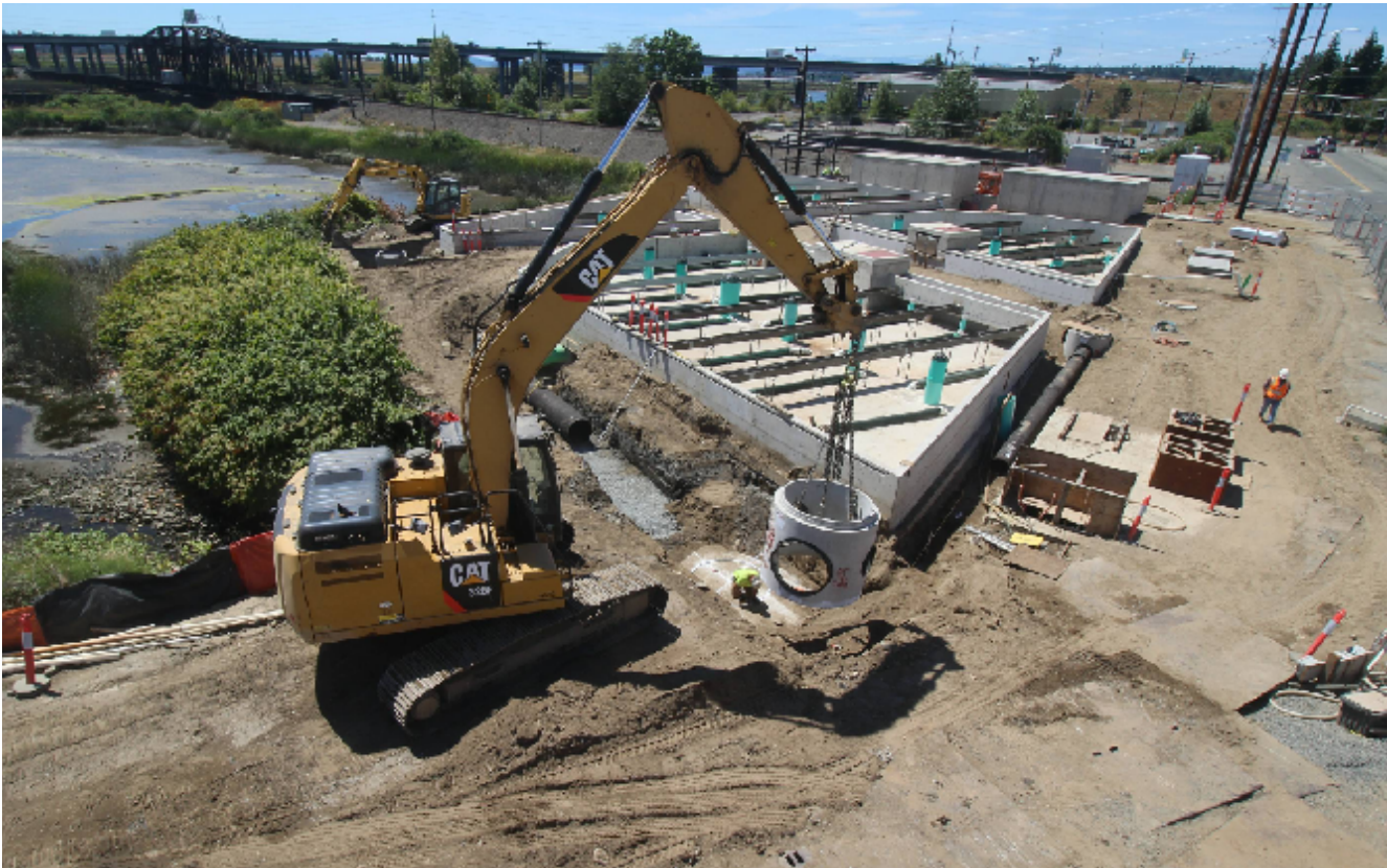
The Downtown Stormwater Treatment Facility pictured under construction in the summer of 2023.
