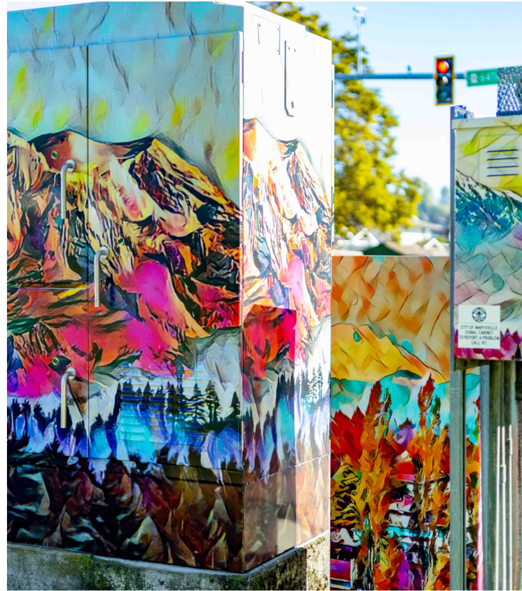
Form and function combine in this decorative traffic signal box. Traffic signal management is an aspect of Transportation System Management and Operations (TSMO), an emerging technology.
