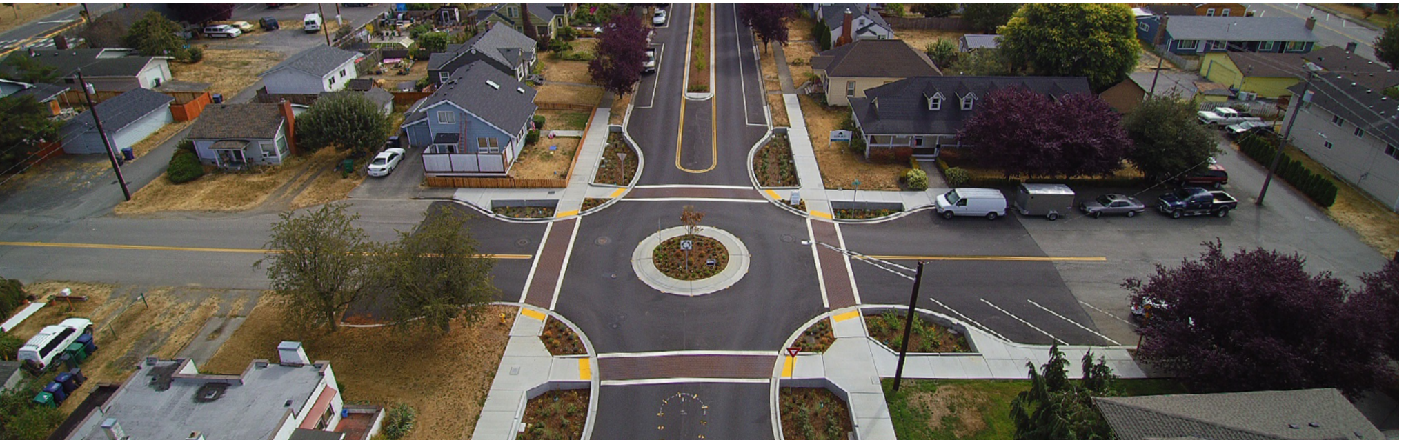
The Third Street Retrofit project enhanced pedestrian safety and water quality while beautifying the Downtown.
