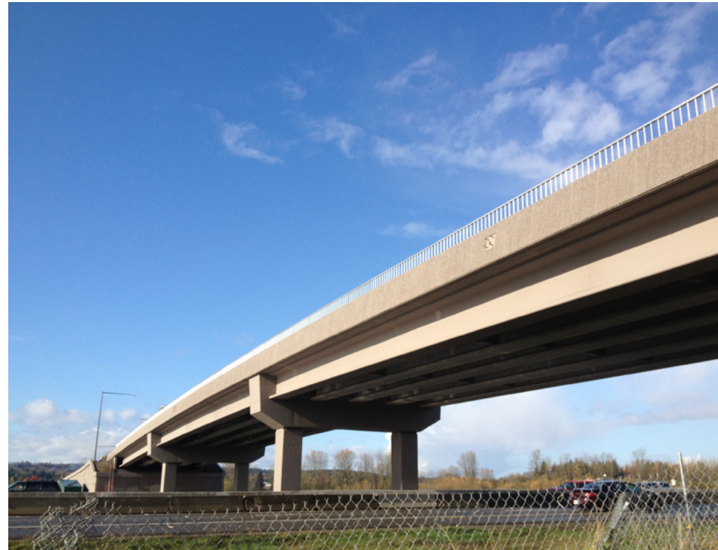
The 156th Street Overpass will be converted into a full I-5 Interchange in the future.
