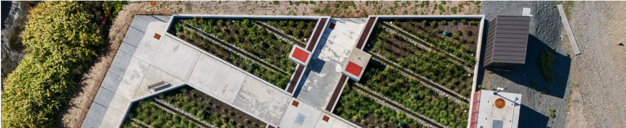
Marysville's Downtown Stormwater Treatment Facility has the capacity to treat runoff from much of the Downtown.
