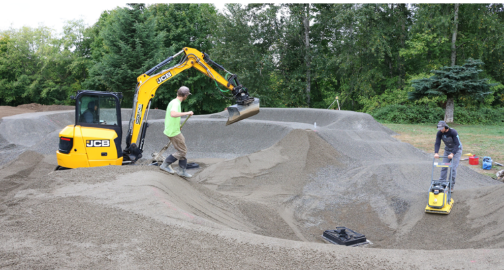
The Parks Division coordinates with Public Works on park maintenance and building new parks such as the Pump Track under construction here.
