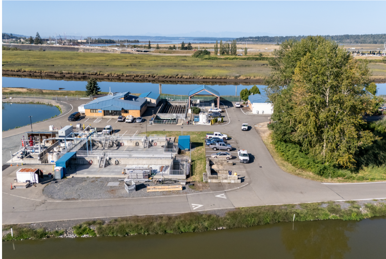
Marysville's Wastewater Treatment Plant ensures that wastewater is properly treated prior to discharge.
