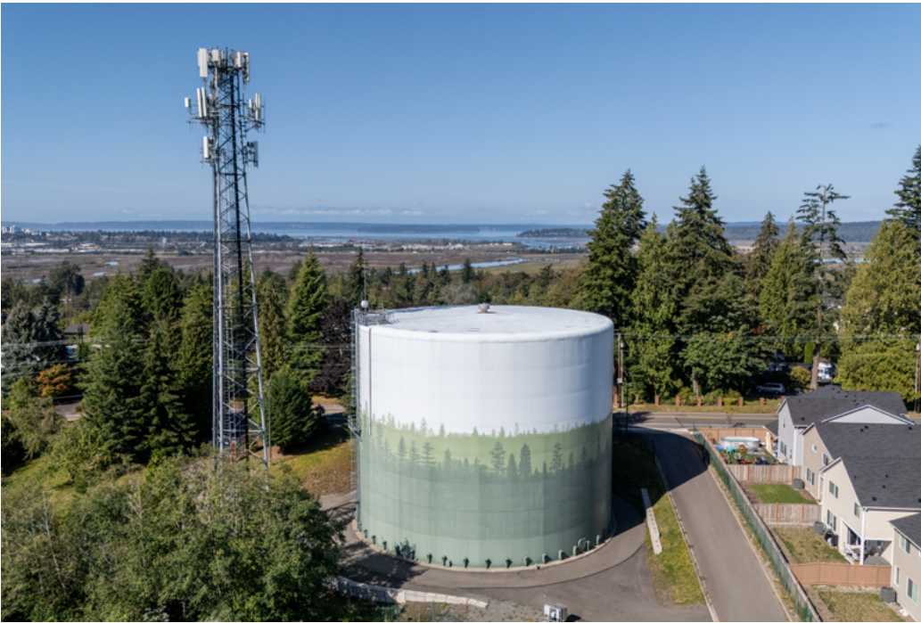
The Sunnyside Reservoir is one of nine city reservoirs that provide a combined total of 24.3 million gallons of water storage for the community.
