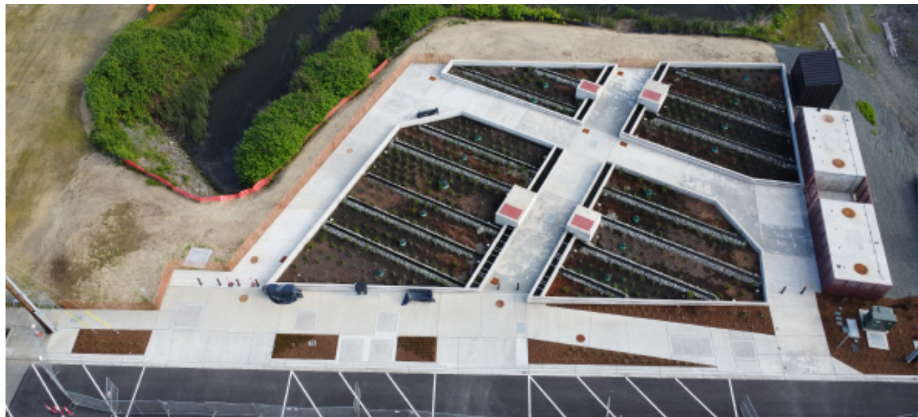
The Downtown Stormwater Treatment Facility treats stormwater from Downtown prior to discharging the clean water to Ebey Slough.
