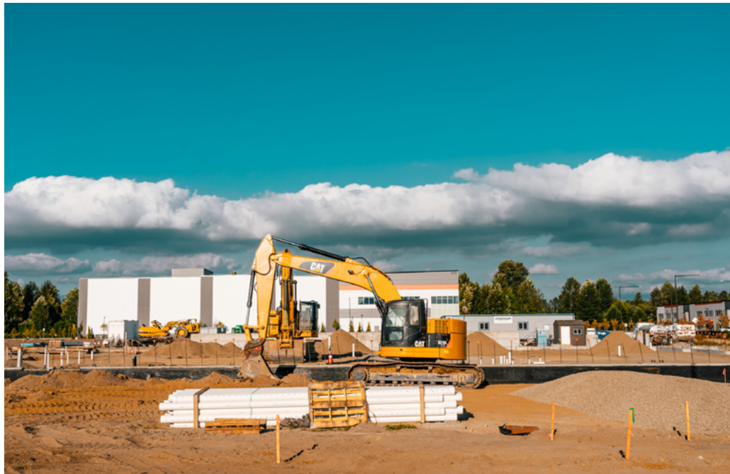
Longstanding plans for a manufacturing and industrial center taking shape in the Cascade Industrial Center.
