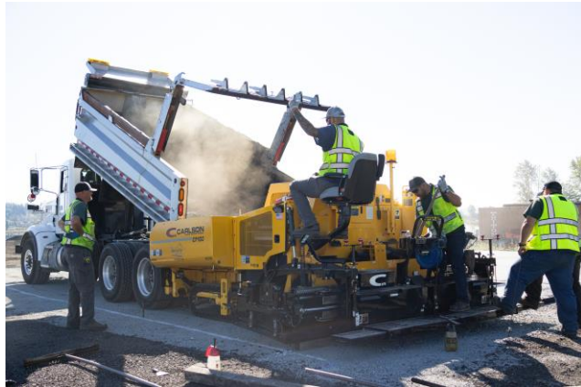
Image 11 Public Works crews working on a road improvement project.
