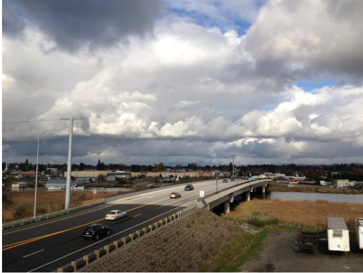
Image 12. A new I-5 interchange is currently being constructed south of Ebey Slough, which will tie into the SR529 bridge shown here.
