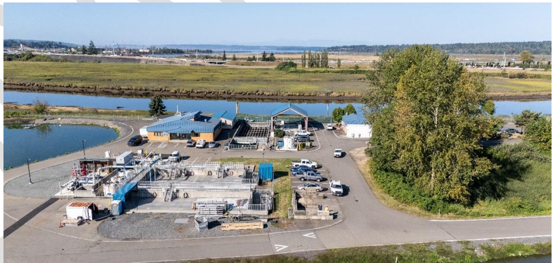
Image 1 Marysville's Wastewater Treatment Plant ensures that wastewater is properly treated prior to discharge.
