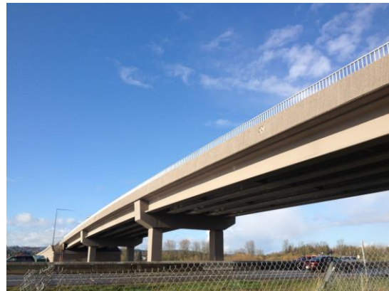
Image 8 The 156 th Street Overpass will be converted into a full I-5 Interchange in the future.
