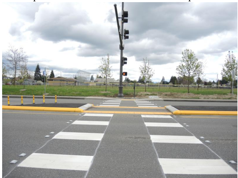
Image 5 The HAWK signal or high-intensity activated crosswalk beacon on 4 th Street enhances safety for pedestrians and bicyclists crossing this busy roadway.
