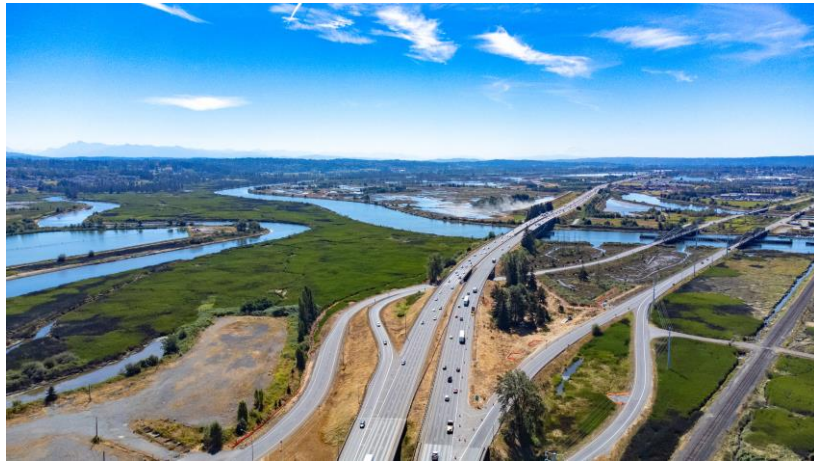
Image 1 Interstate 5 and SR529 are state highways providing vital regional connections.
