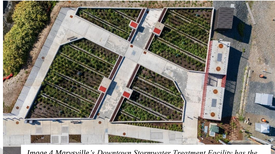
Image 4 Marysville's Downtown Stormwater Treatment Facility has the capacity to treat runoff from much of the Downtown.
