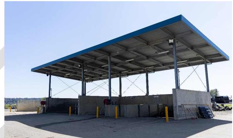
Image 3 The Marysville Decant Facility ensures that stormwater waste can be processed, treated, and disposed of in an environmentally sensitive manner.
