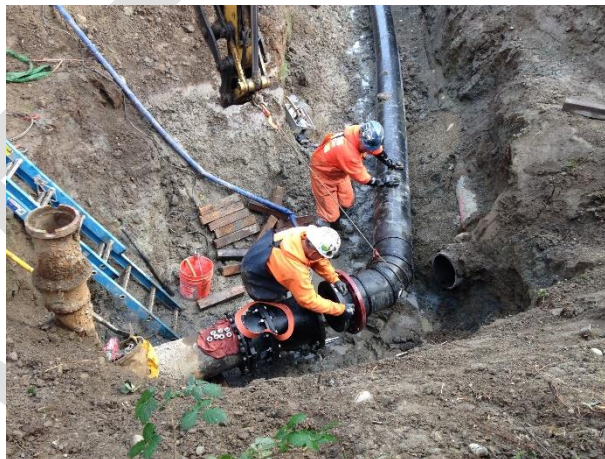
IMAGE 6 Workers maintain a utility line. This is a placeholder; PSE specific photos have been requested.
