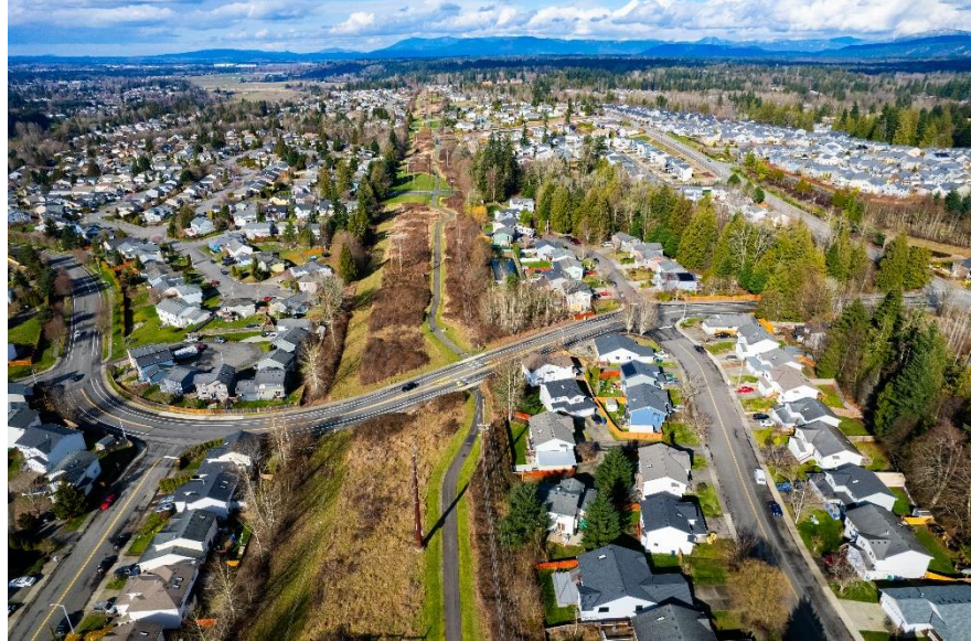
IMAGE 7 The Olympic Pipeline, Puget Sound Pipeline, and other major regional utilities, are located in the utility corridor shown here.
