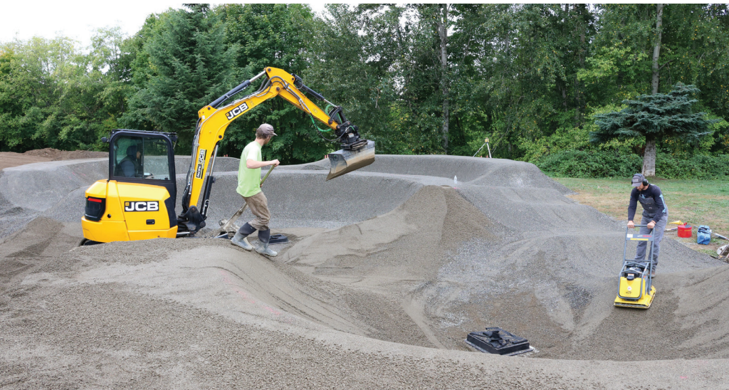
The Parks Division coordinates with Public Works on park maintenance and building new parks such as the Pump Track under construction here.
