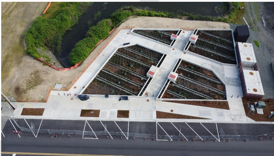
IMAGE 1 The Downtown Stormwater Treatment Facility treats stormwater from Downtown prior to discharging the clean water to Ebey Slough.
