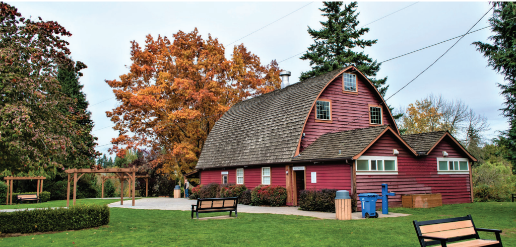
The Jennings Parks Barn is used for various events and also offers restrooms for park visitors.
