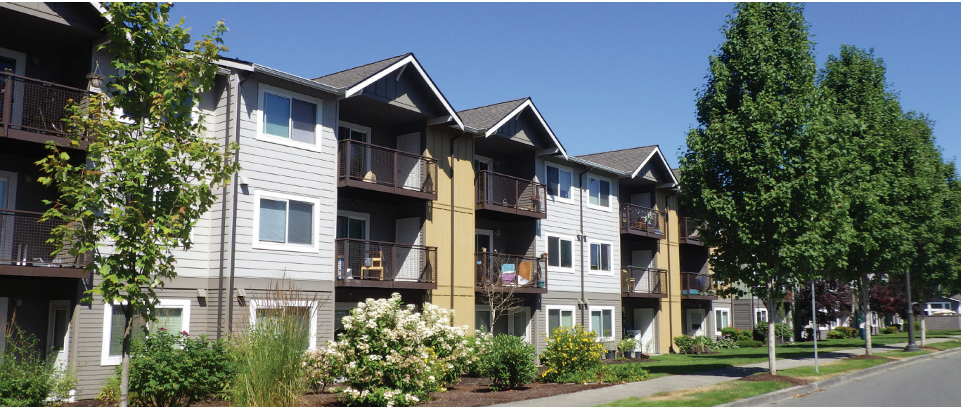
Streets trees, landscaping, and private balconies enhance the quality of life for residents of this multi-family residence.
