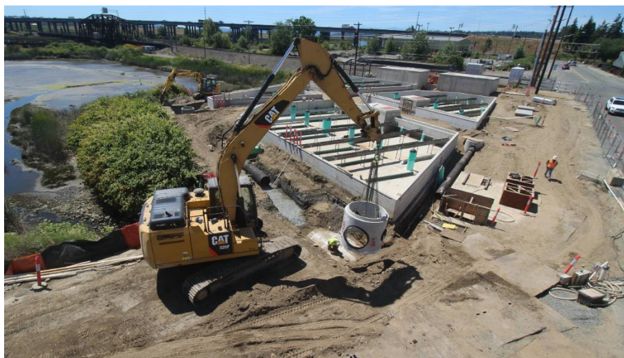
IMAGE 3 The Downtown Stormwater Treatment Facility pictured under construction in the summer of 2023.
