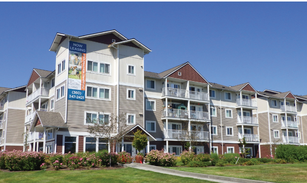
The Vintage at Lakewood, is an apartment that provides affordable housing for seniors.
