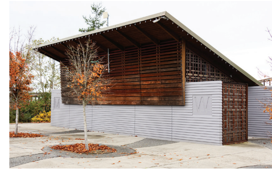
Restrooms at the Ebey Waterfront Park.
