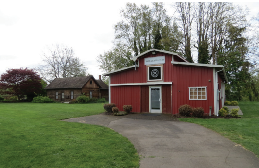
Rotary Ranch, in Jennings Memorial Park, is used for recreational services.
