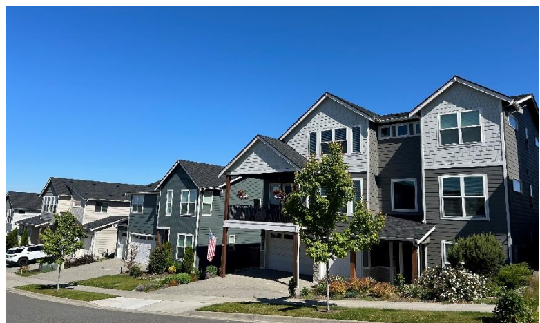
Image 33 New residences in the Sunnyside Neighborhood have typically included traditional gables, with those along Sunnyside Boulevard often taking advantage of the expansive westward views.
