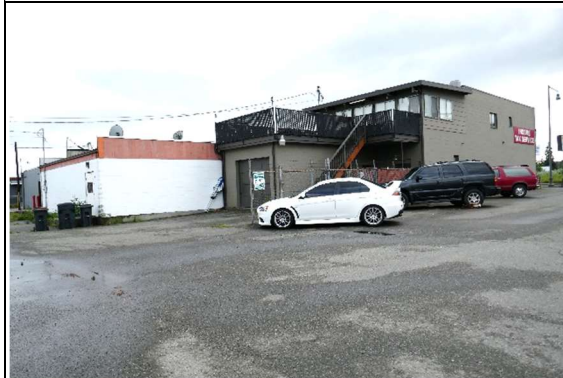
Looking SW at rear of property
