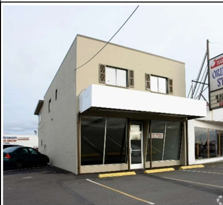
Looking E from State Ave
