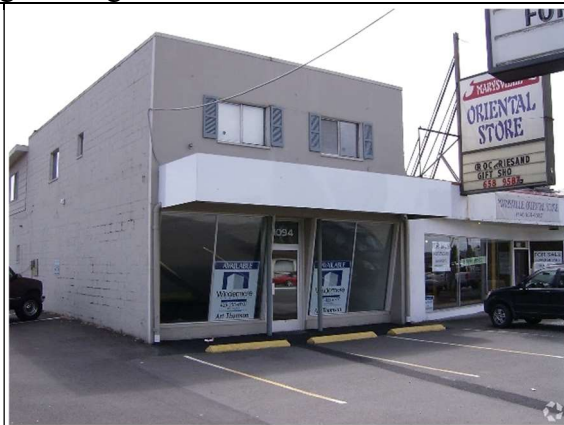
Looking E from State Ave
