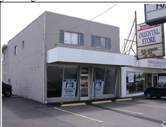
Looking E from State Ave
