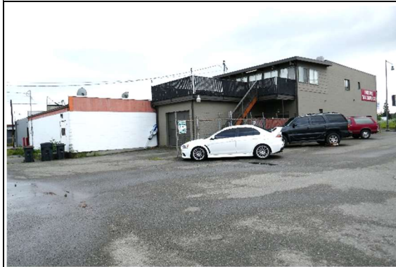
Looking SW at rear of property
