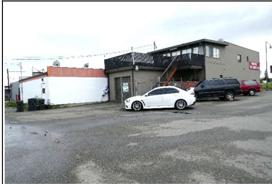
Looking SW at rear of property
