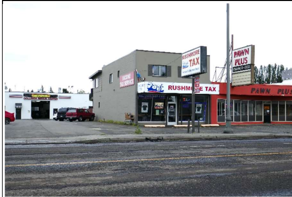
Looking E from State Ave
