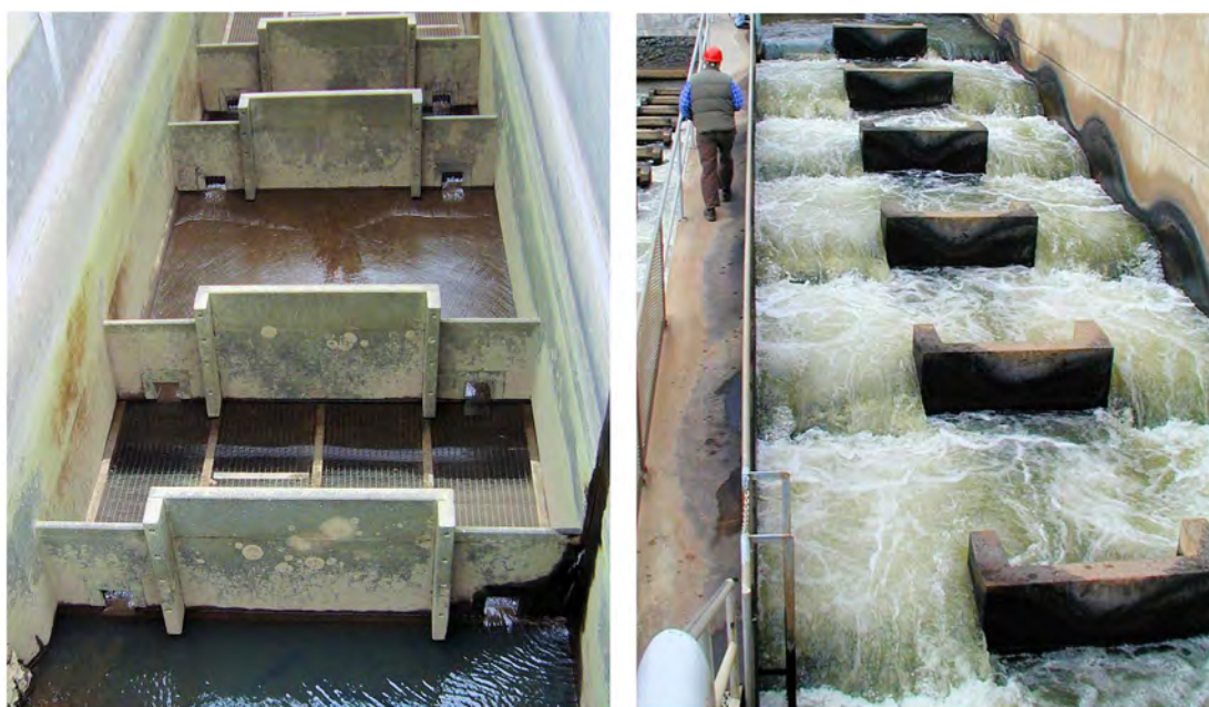
(a) Looking downstream
